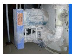
Corrosion-resistant shafts are used to eliminate the need for shaft sleeves. Impellers are keyed to the shaft, providing a secure fit and protection, should momentary reverse rotation occur. The swing-out mount is a popular optional feature allowing easy inspection of the pump and quick access to the tank interior.
